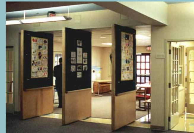
5 Full height pivoting panels are used to open or close off space
