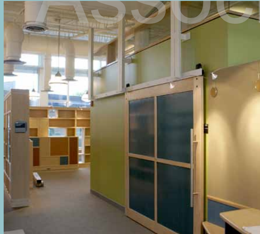
3 Barn style doors and hardware utilized to close off or create large openings
